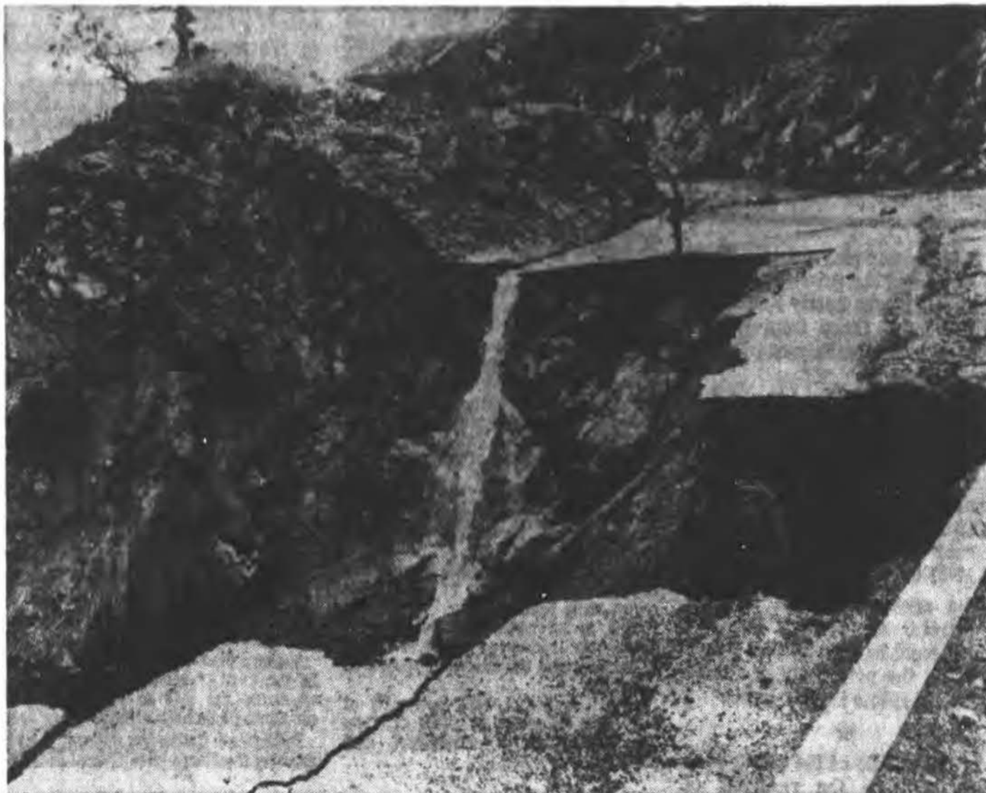
WATERFALL TUMBLES DOWN CANYON WHERE BIG TUJUNGA CANYON ROAD ONCE RAN. Large Section of Road Collapsed as Result of Nine Days of Rain in Southern California
