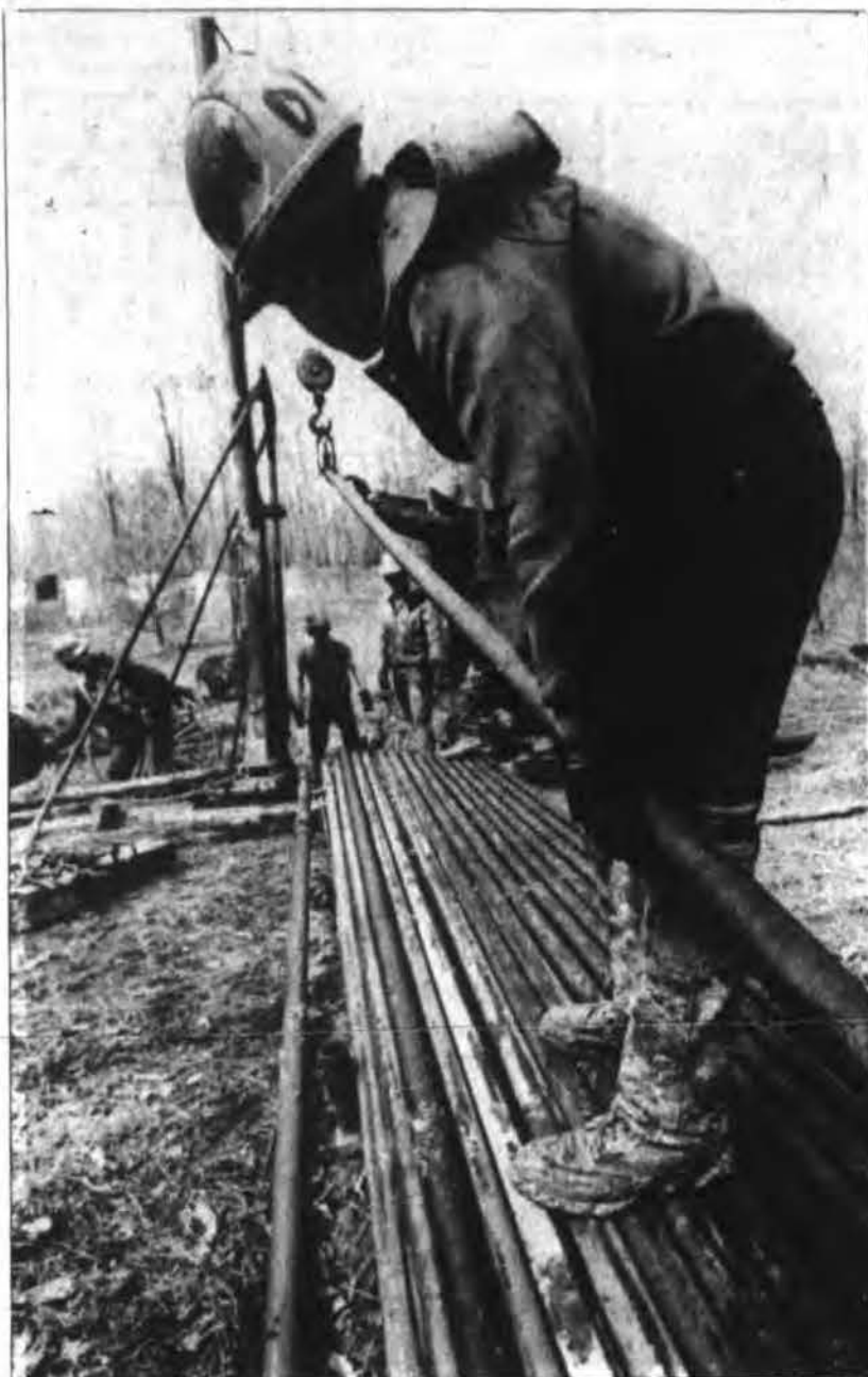
Leo Munday steadies a section as classmates check for leaks in piping pulled from one of Bradford Area High School's oil wells.
